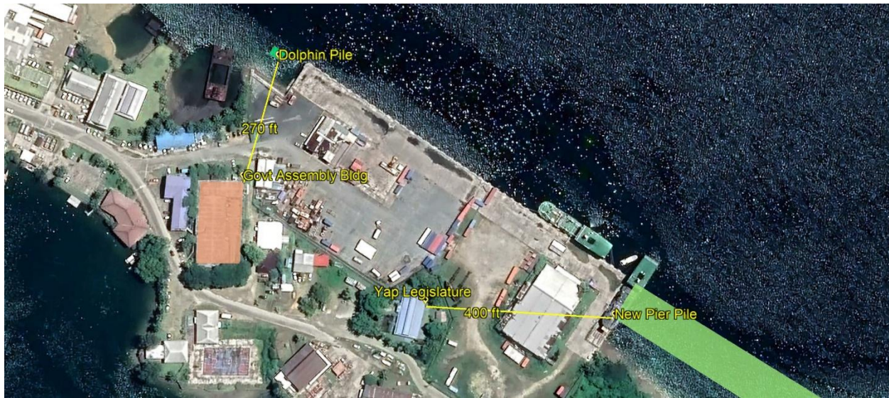
Figure 3: Seaport Construction Activity Areas
